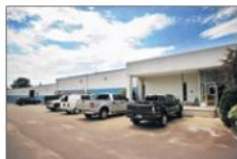
Advanced Grow Labs medicinal marijuana growing facility being constructed at 400 Frontage Road in West Haven.
